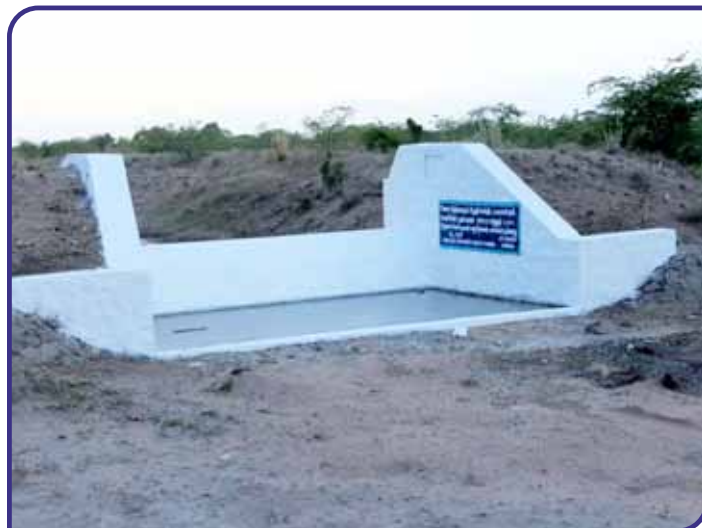
Check-Dam Construction in A. Lakshmiapuram Village
