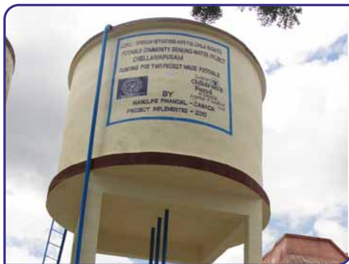
Water Tank Construction in Chellaiapuram Village
